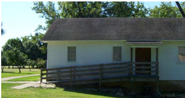
Cooperage Museum accessible entrance
