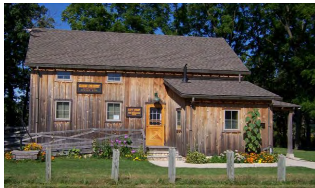
Visitors Center (ramp entrance on left and restroom path on right)
