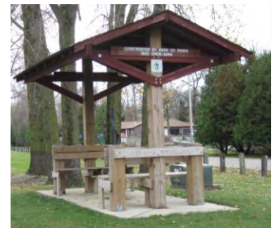
Well shelter (no accessible route)
