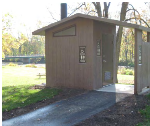
Accessible restroom and route
