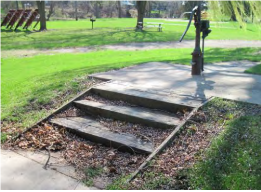
Stairs from shelter to well
