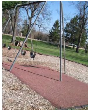
Poured in place surface
