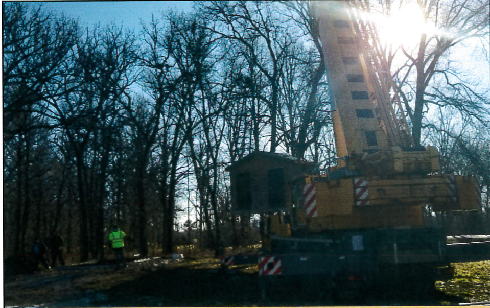
Happy Hollow Restroom Install
