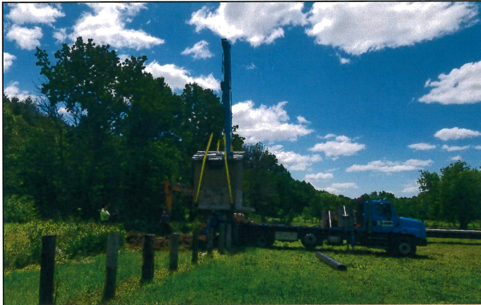
Gibbs Lake Restroom Install
