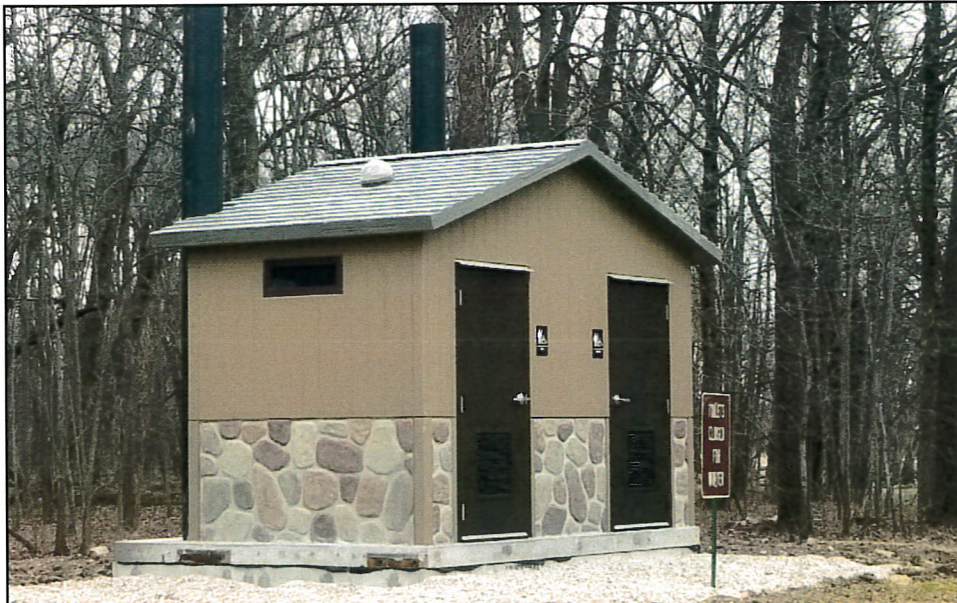
Happy Hollow Restroom
