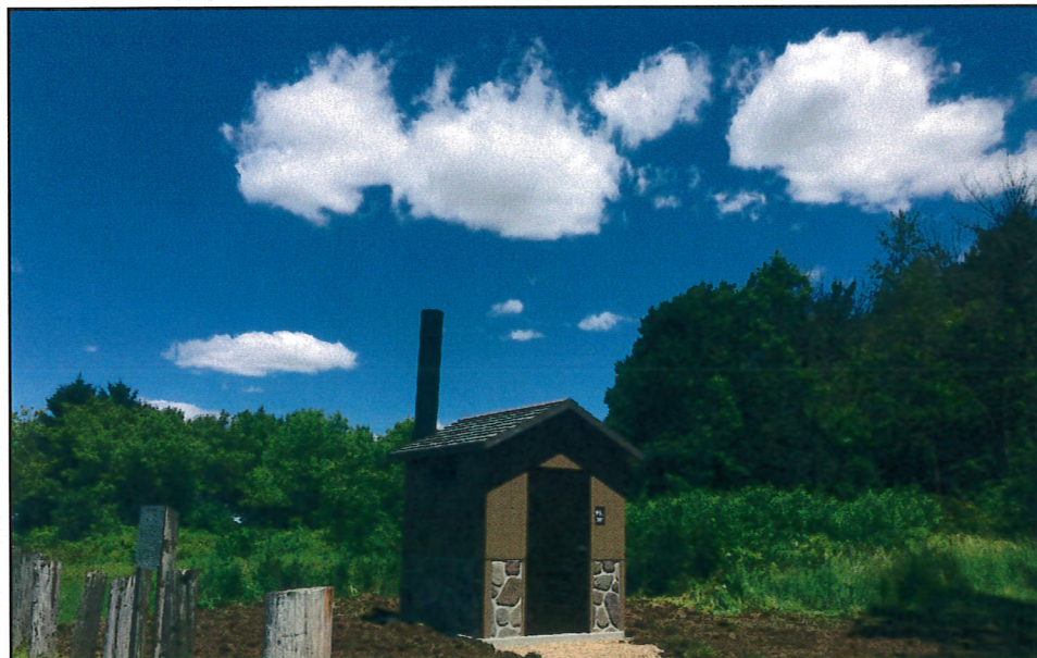
Gibbs Lake Restroom
