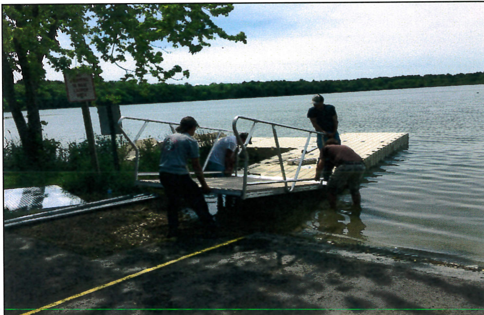
Gibbs Lake Boat Launch Installation
